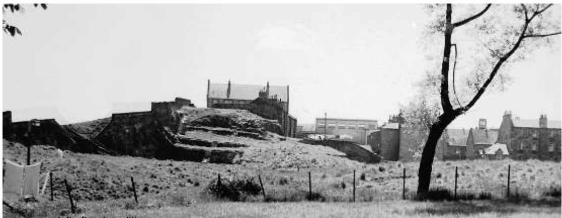
Empty space left after demolition
